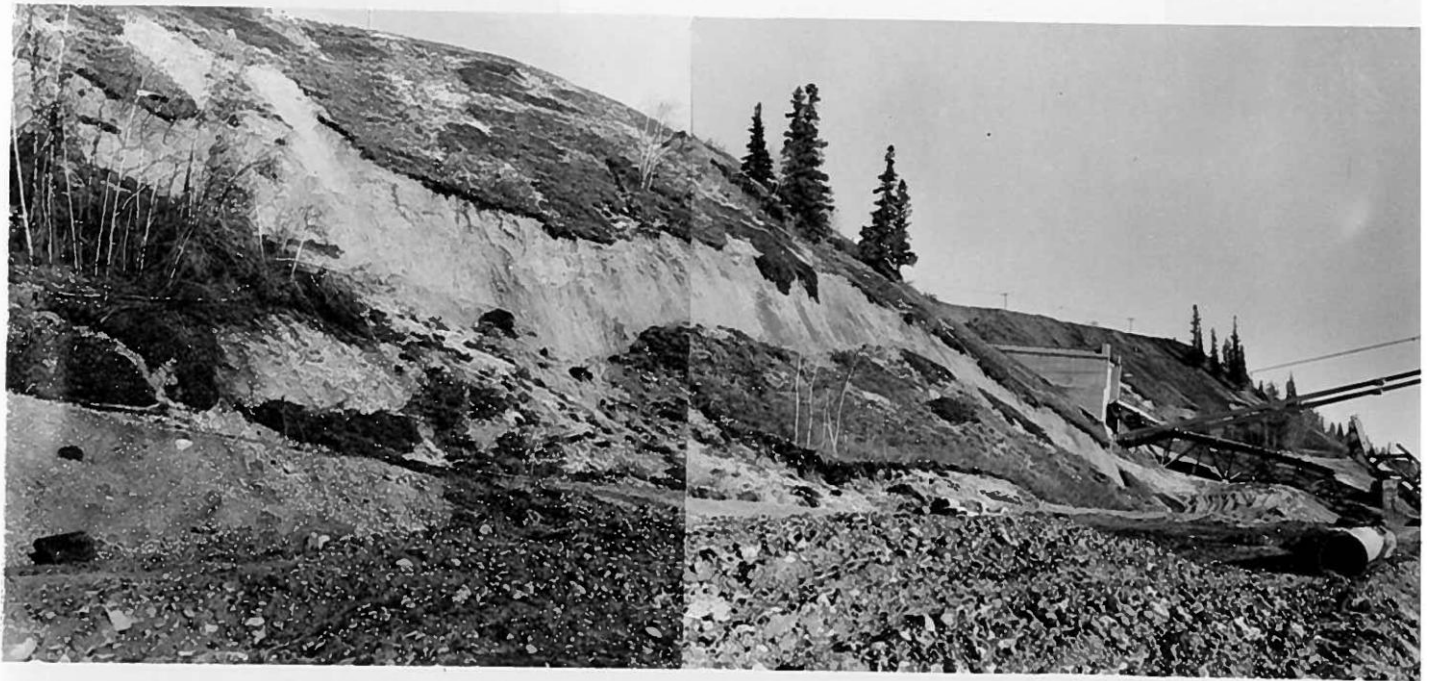
Figure 3. View from west of scarp of landslide, North abutment and collapsed approach span in background
